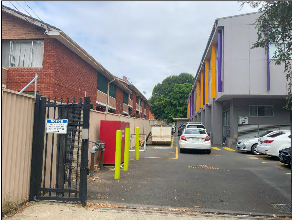
Figure 19: Southern part Rissalah College, which is directly to the east of the subject site
