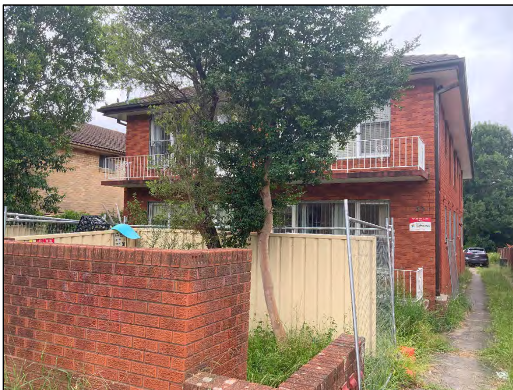
Figure 4: Front of the existing building on the subject site
