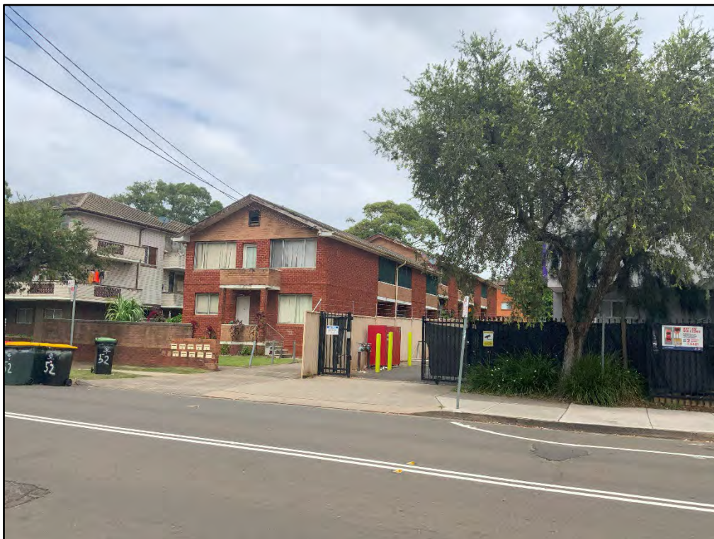
Figure 22: Residential flat building at 52 Hampden Road, southeast of the subject site
