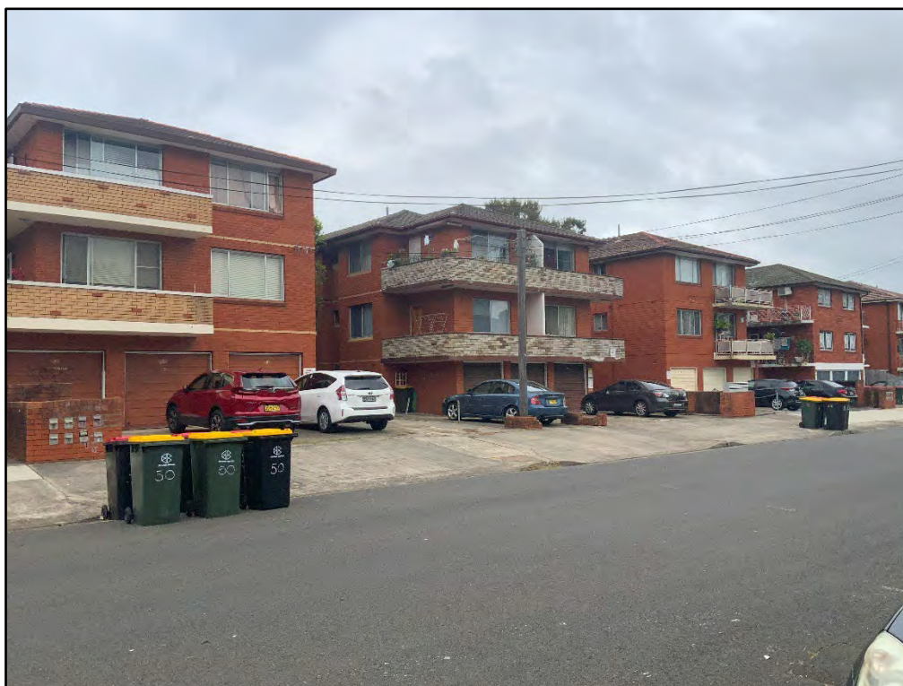
Figure 35: Residential flat buildings opposite the subject site on the western side of MacDonald Road, looking southwest from the subject site
