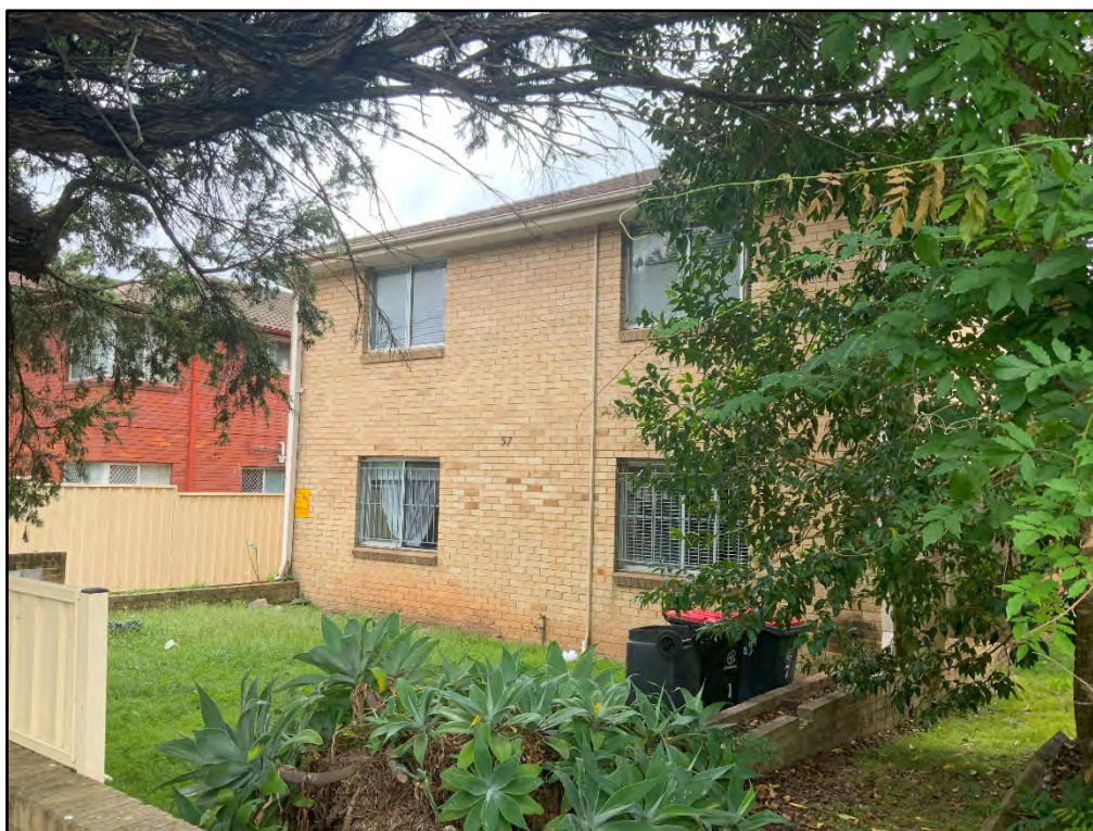
Figure 11: Front of the residential flat building adjoining the subject site to the north
