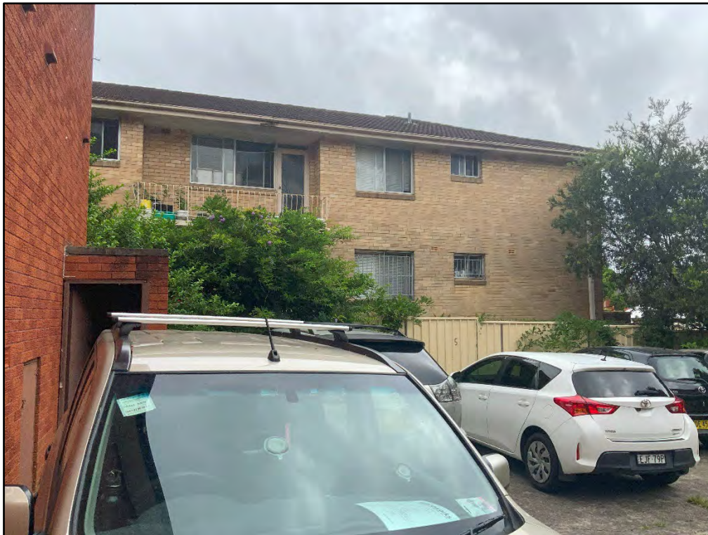
Figure 15: Interface of the subject site and the adjoining residential flat building to the north
